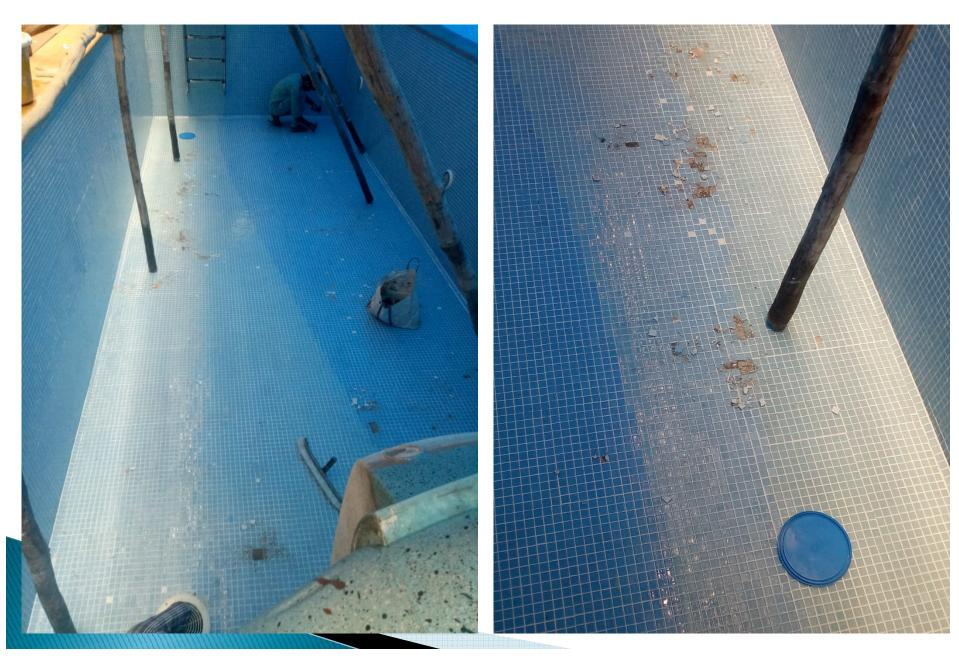
Damaged glass tiles refixing, Epoxy Grouting and Cleaning Work.
