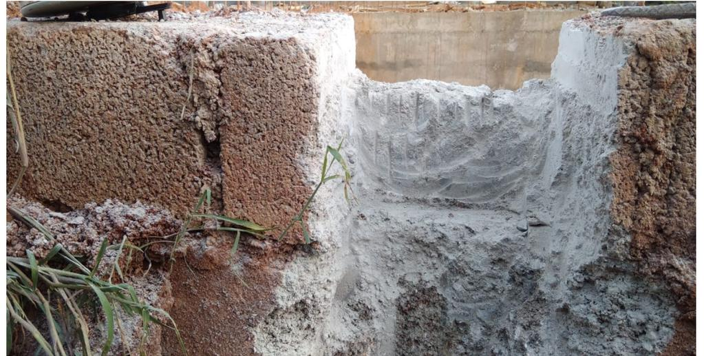
Swimming Pool Shell Construction & wall cutting to fix Skimmer Boxes
